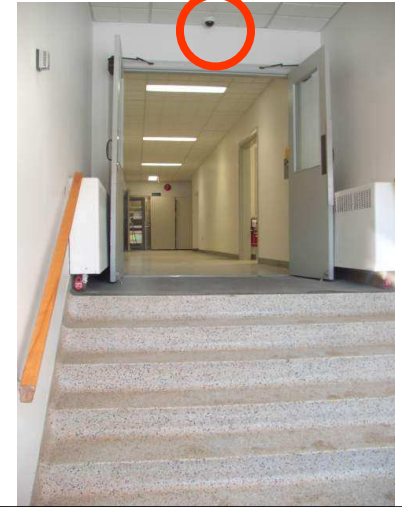
Indoor w/o sunlight, CCTV
